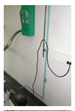
The service disconnect switch for the RF furnace is the green box on the wall. In order to turn the furnace on, the water pump (which supplies cooling water to the leads and coil) must be plugged in (no switch) and the flow valve opened.
