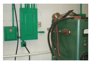
The copper terminals on the right (at left, above) and left (at left, below) sides of the RF generator power supply are live and dangerous. DO NOT TOUCH, the voltage and current are well beyond lethal! Advise students of the hazard at the beginning of the class.
